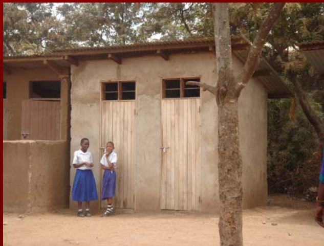
A relatively nice example of pit latrines in a primary school (all things being relative)
